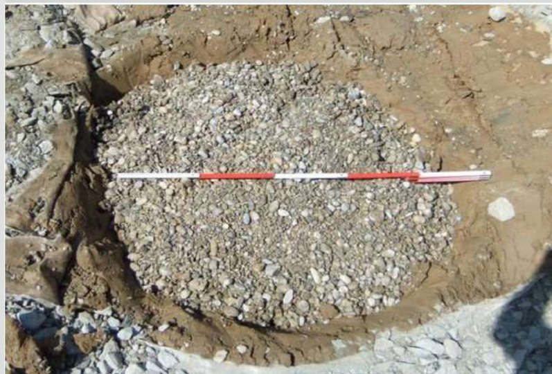
Fig. 14: "Head" of a vibrodisplacement stone column
