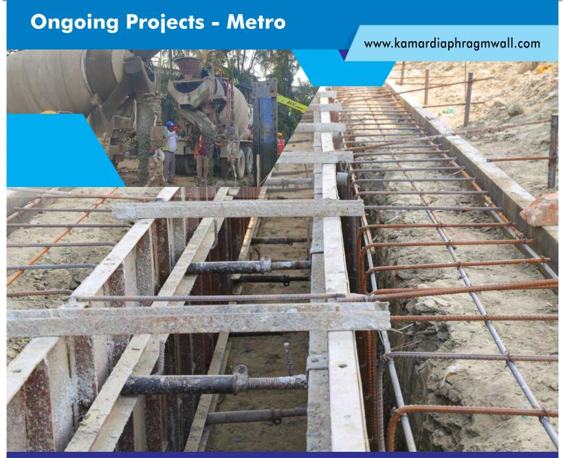
Construction of Diaphragm Wall 600 mm width for RRTS Project, Dwarka, Delhi.
