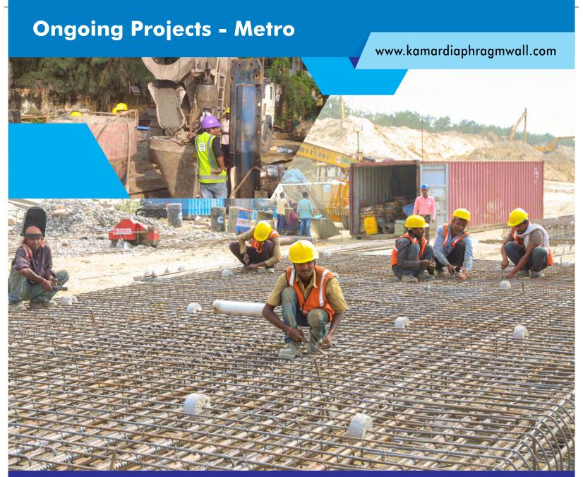
Construction of Diaphragm Wall 1000 mm, 800 mm & 600 mm width for Kapodra, Central Warehouse & Labeshwar Station, Surat, Gujarat.
