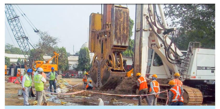
Diaphragm walls are particularly suited to the construction of very deep retaining walls and often seen together with 'top down' construction techniques. These allow building work to take place above ground, while deep excavation work continues at the same time. Diaphragm walls generally provide a high level of leak protection to deep foundations.
