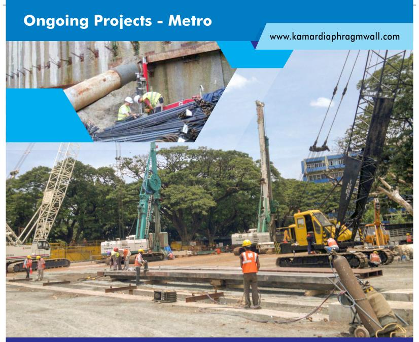
Construction of Diaphragm Wall 1000 mm & 800 mm width for Naya Ganj Station, Kanpur Metro, Uttar Pardesh.
