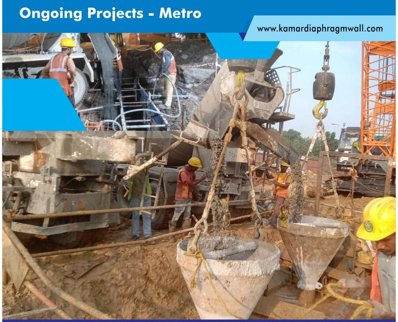
Construction of Diaphragm Wall 1200 mm width for Maskati Metro Station, Surat Metro.
