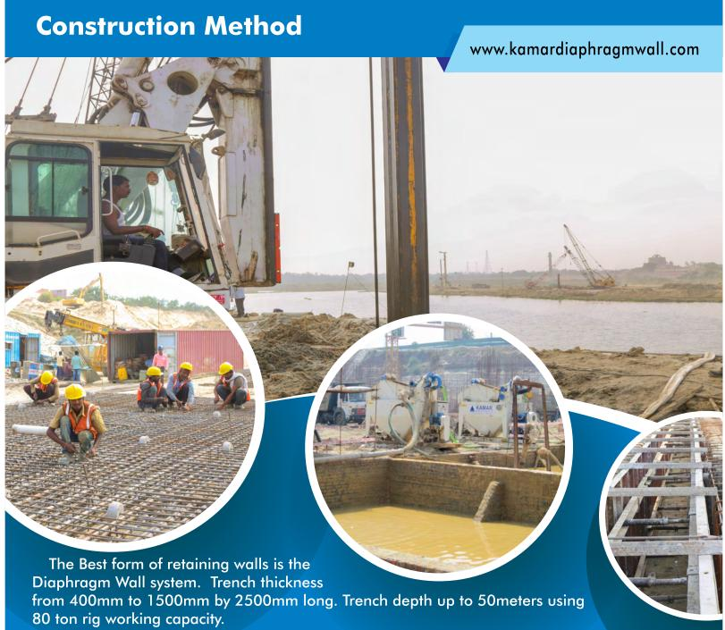
Diaphragm Wall is a cast in place with a reinforced or plain concrete retaining wall constructed by special designed trench equipment with multiple drill head or clamshell bucket. Diaphragm walls are underground structural elements commonly used for retention systems and permanent foundation walls. They can also be used as deep groundwater barriers The specialty in this method is to apply stabilizing fluid (bentonite slurry or polymer slurry) for preventing collapse of excavated trench.
